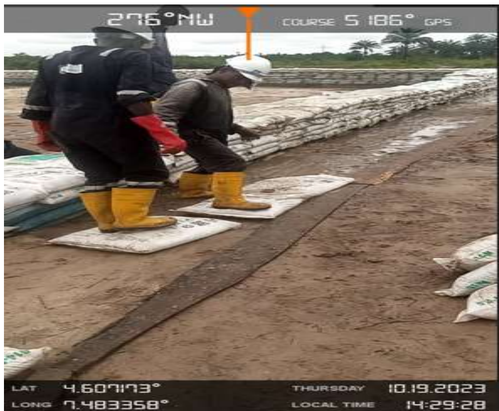
Plate 2: Stabilizing of Sandbags Laying
