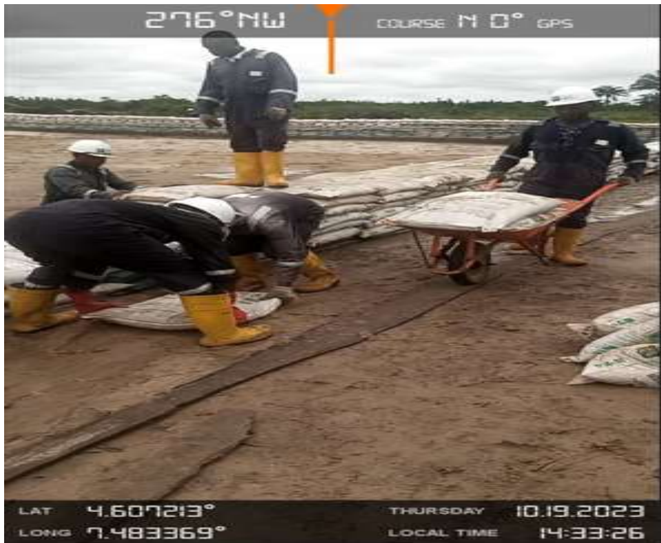
Plate 5: Cross Section of Stacking Sandbags Ongoing
