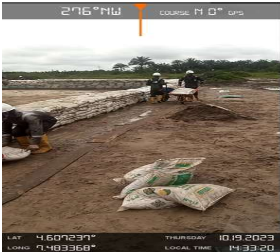
Plate 6: Stacking of Sandbags Ongoing
